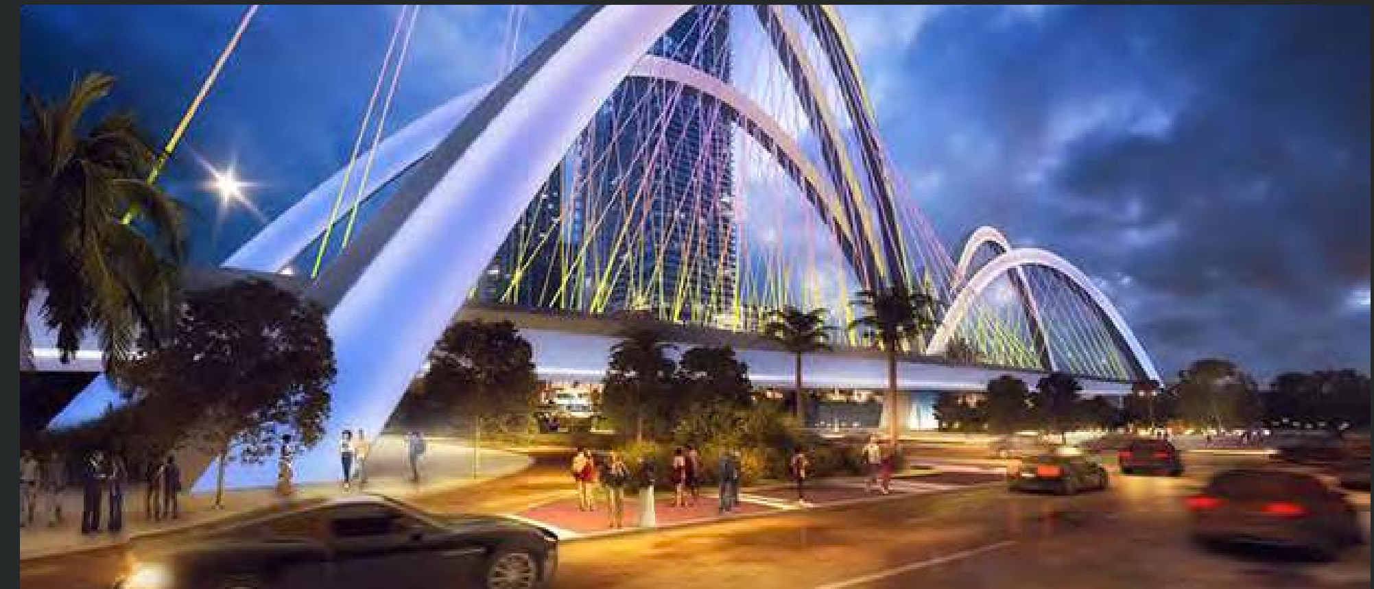
I-395 SIGNATURE BRIDGE
